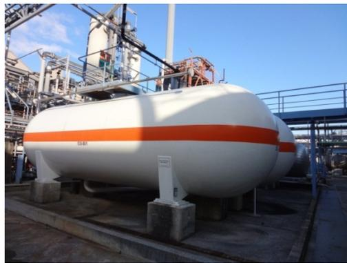
**Figure 1: Horizontal cylindrical reservoirs resting on four legs system support.**
