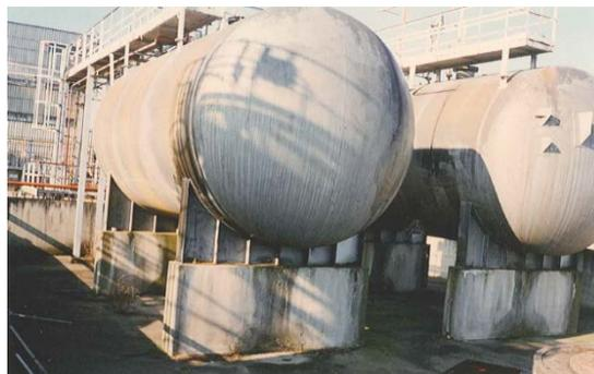
**Figure 2: Horizontal cylindrical reservoirs resting on saddles of support.**
