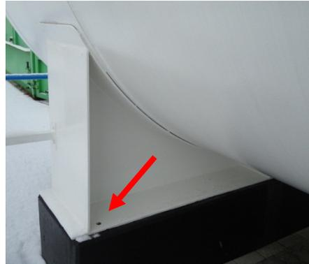
**Figure 3: Horizontal cylindrical reservoirs resting on saddles.**
